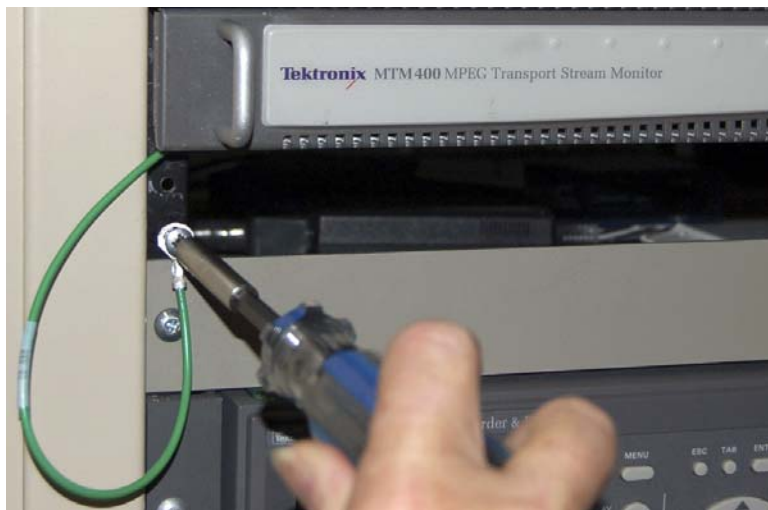
Figure B-5: Attaching the ground strap to the rack frame
